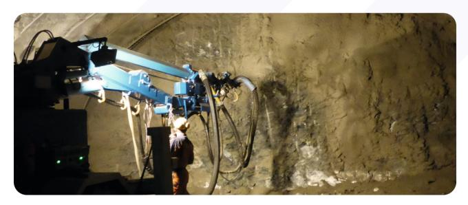
Sprayed concrete applications must ensure safety and be formulated to last. Master Builders Solutions® offers a wide range of admixtures for addition during concrete batching and on-site.
