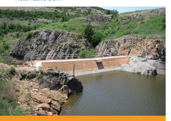
Ketch Lake Dam, built by the landowner Frank Ketch in the 1930's, was built of cobblestone and was a stock pond for cattle. Subsequently, it became a recreational pond. When the dam started giving way in 2010, the Army Corps of Engineers decided to build a new dam directly behind the existing dam. The new dam is 36 feet (11 m) high, 140 feet (43 m) wide and 6 feet (1.8 m) thick at the top and 80 feet (24 m) wide and 20 feet (6 m) thick at the bottom.
